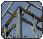
STEEL FRAMING CONTRACTORS
